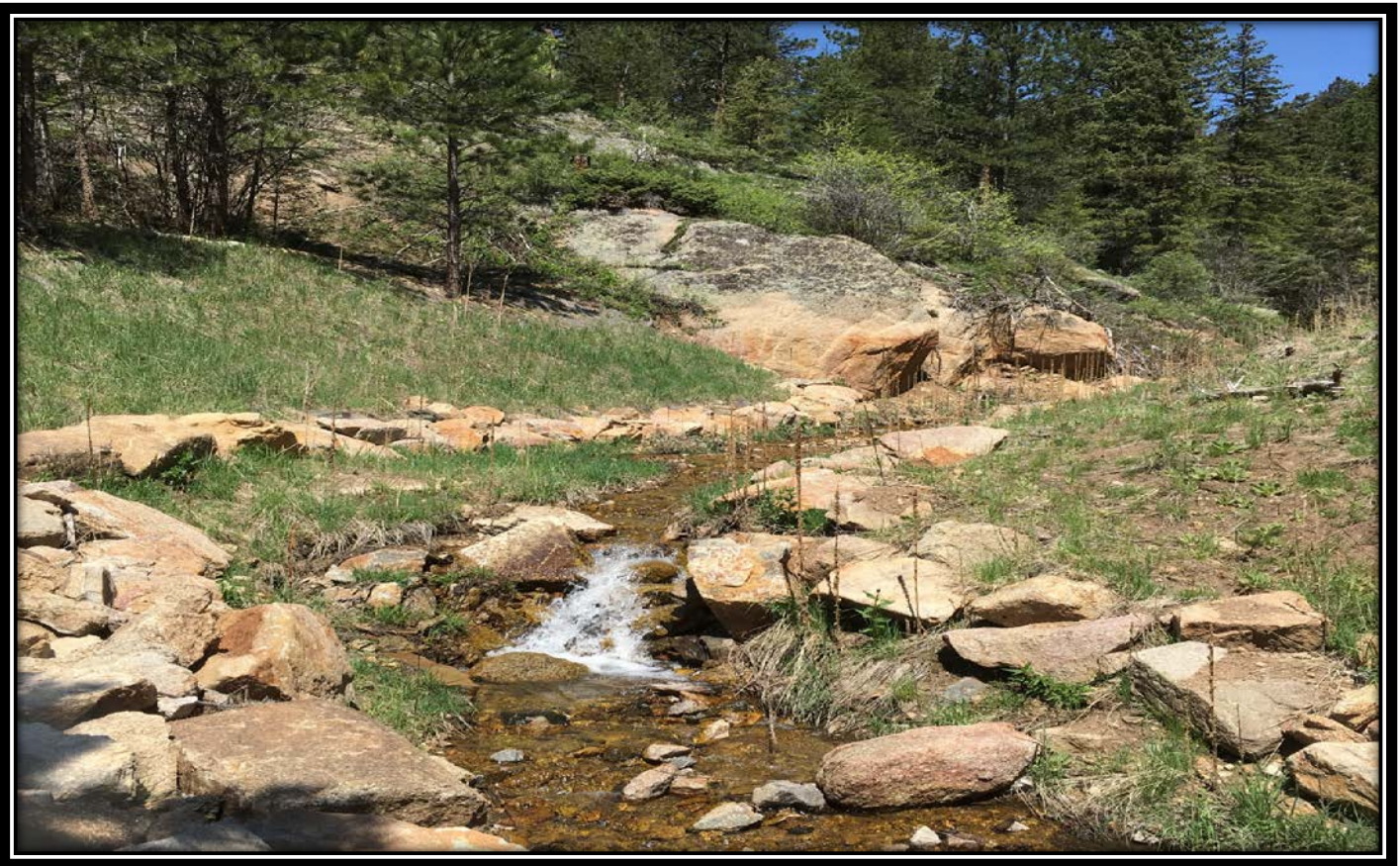
Photos #12 and #13 - Reclaimed Cut Bank Slopes
