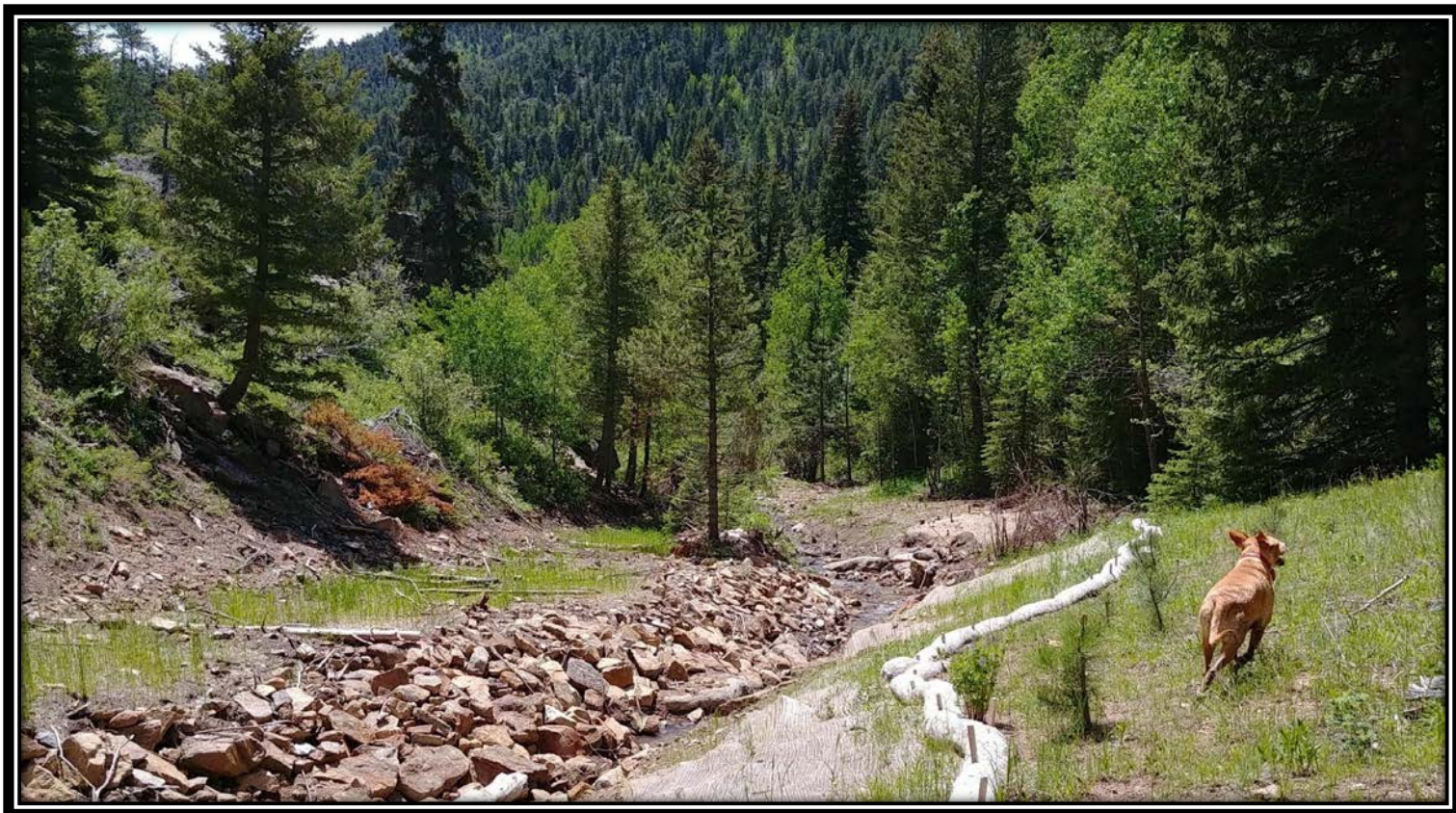
Photo #22- One Year Post Reclamation - Reclaimed and Revegetated Repository- Armored on Both Sides of Channel and Topsoil Cap
