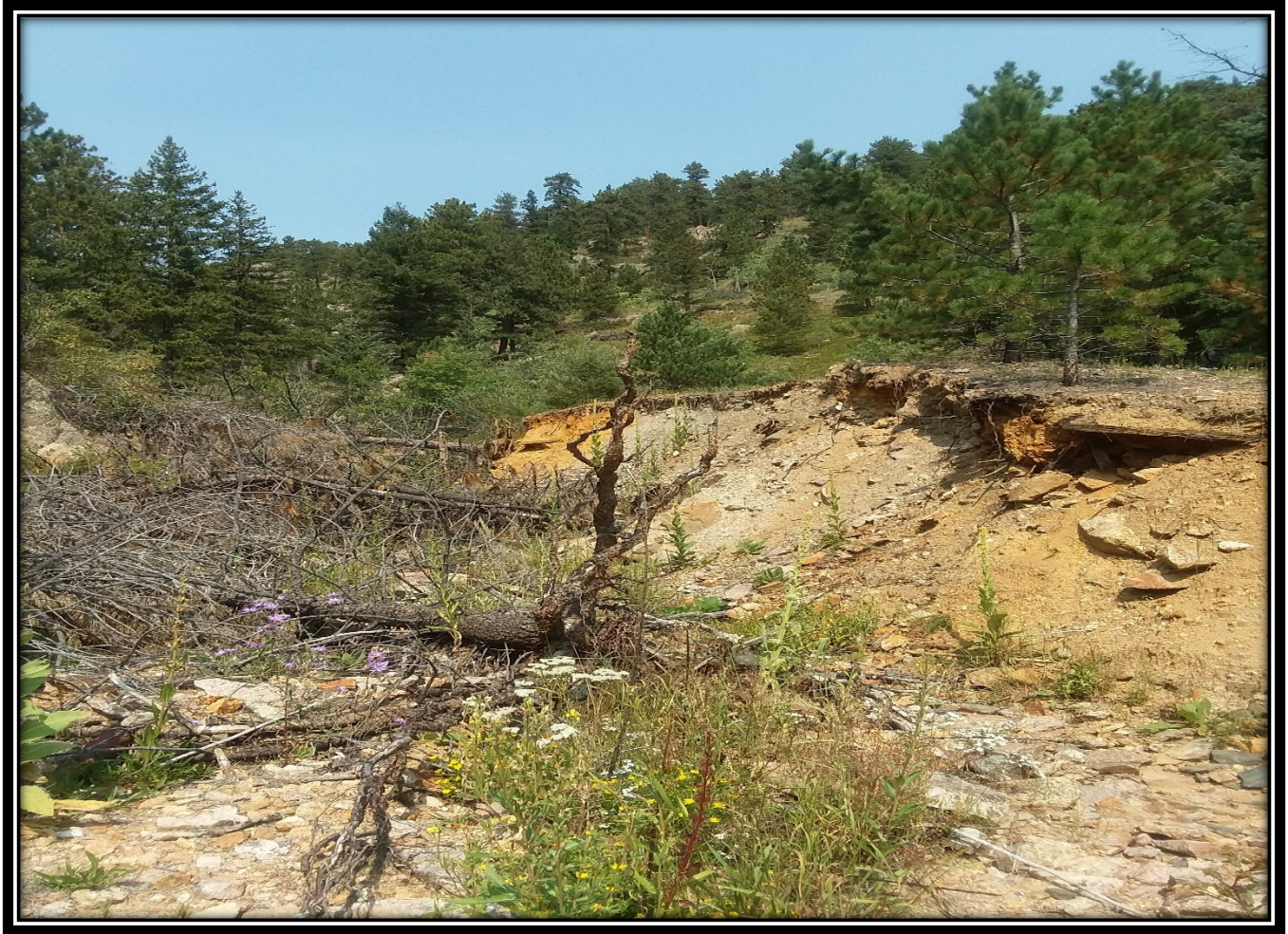
Photo #1-Cut Bank Slopes containing Radioactive Metal- Laden Waste Rock/Wooden Debris Deposited by Flood Pre-Reclamation
