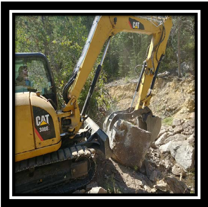
Photo # 6-Armoring the Channel with Riprap
