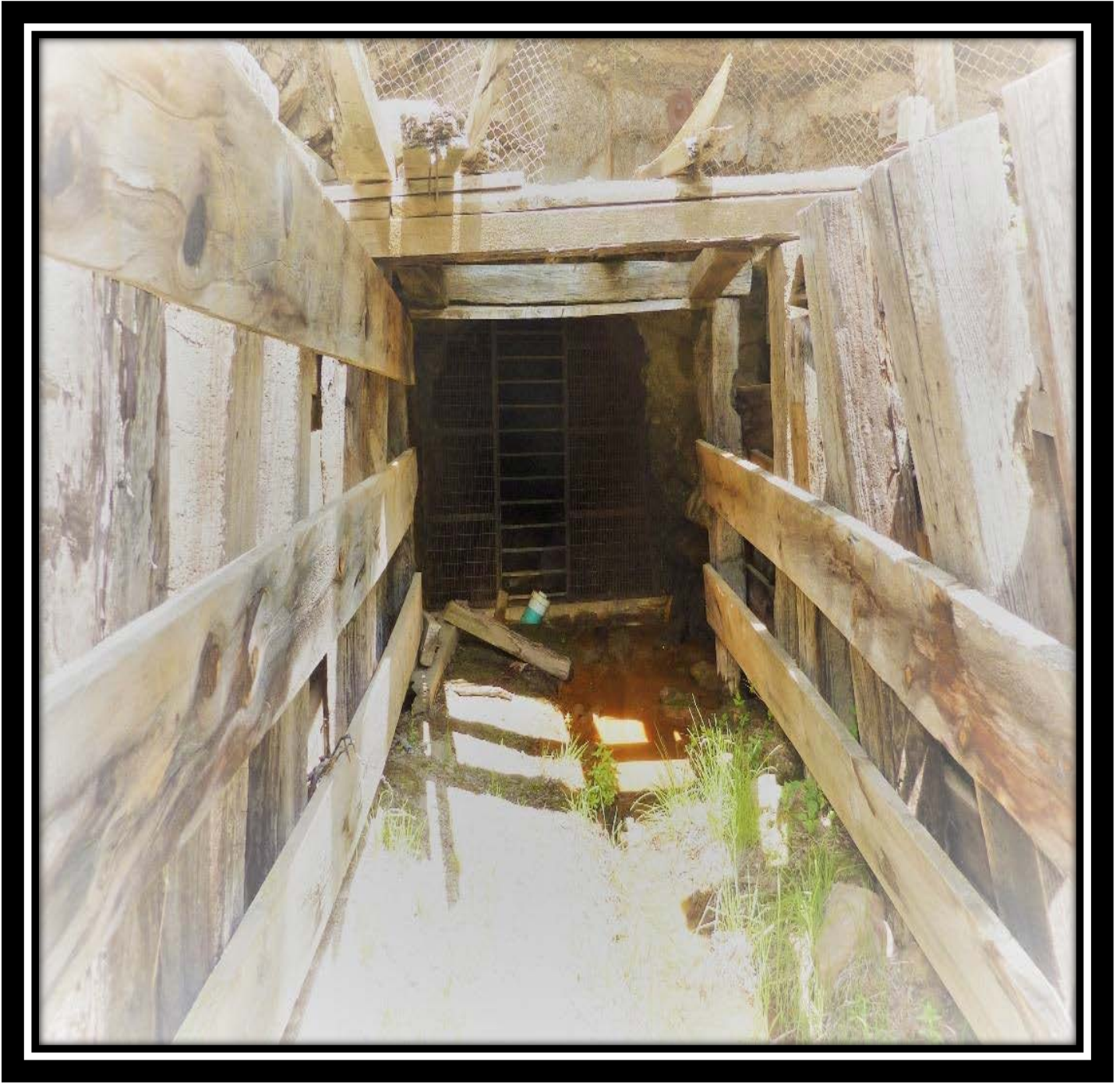
Photo #21-Mine Portal Safeguarded with Bat Grate
