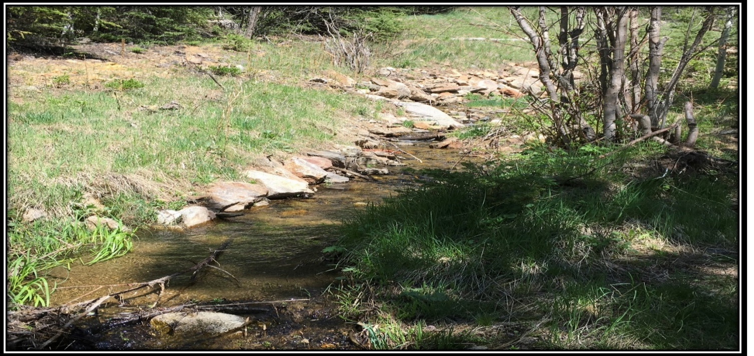
Photos # 17 and #18 - Toe of Existing Repository -Pre and Post-Reclamation
