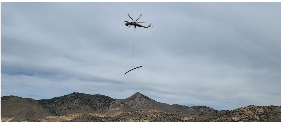
Off-site construction materials transported to site via air crane with respect to cultural and historical sensitivity.
