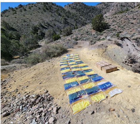
Examples of closure methods used to avoid the use of historic waste rock piles. Shaft sealed with polyurethane mine foam to prevent settling. Concrete pumps were used for footing construction to comply with access restrictions.
