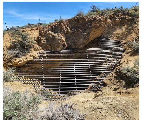
Incline bat-compatible closure.
