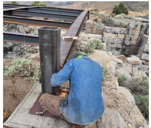
Cupola construction of footings and floor, with all footings dug completely by hand. Use of mechanized equipment was prohibited due to cultural concerns. All footing concrete was tested to ensure 4000 psi break strength. Evidence of epoxy before being inserted in Bedrock.
