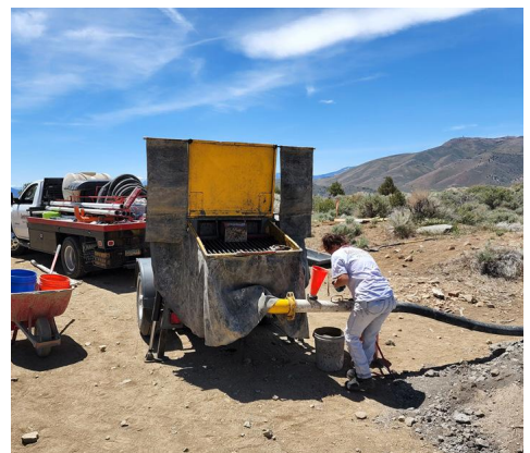
Examples of closure methods used to avoid the use of historic waste rock piles. Shaft sealed with polyurethane mine foam to prevent settling. Concrete pumps were used for footing construction to comply with access restrictions.
