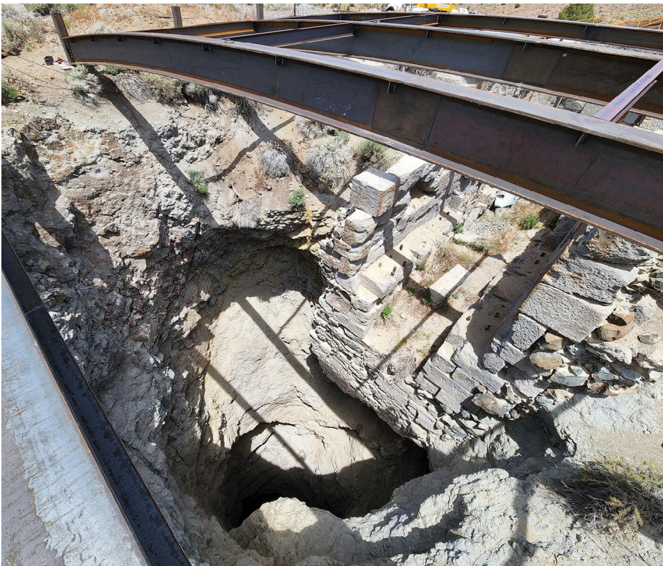
Beams span the Forman Shaft, 165 ft. deep during construction.
