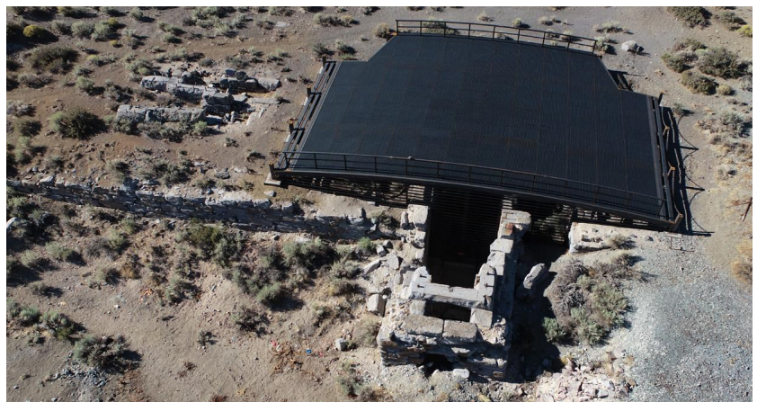
Aerial view of (the largest known) completed wildlife-compatible cupola.
