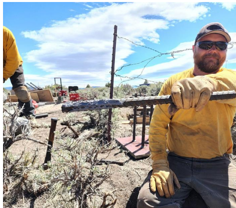
Cupola construction of footings and floor, with all footings dug completely by hand. Use of mechanized equipment was prohibited due to cultural concerns. All footing concrete was tested to ensure 4000 psi break strength. Evidence of epoxy before being inserted in Bedrock.
