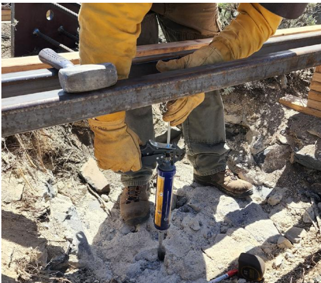
Cupola construction of footings and floor, with all footings dug completely by hand. Use of mechanized equipment was prohibited due to cultural concerns. All footing concrete was tested to ensure 4000 psi break strength. Evidence of epoxy before being inserted in Bedrock.
