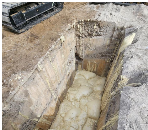
Examples of closure methods used to avoid the use of historic waste rock piles. Shaft sealed with polyurethane mine foam to prevent settling. Concrete pumps were used for footing construction to comply with access restrictions.
