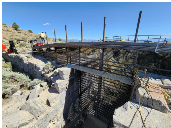
Front view of cupola gate under construction by EPS.
