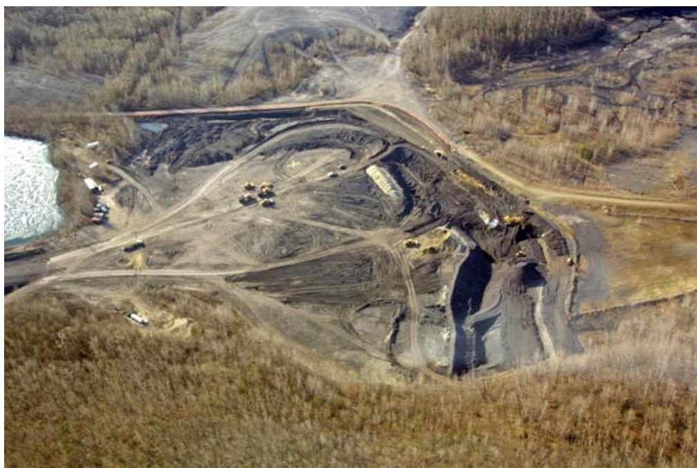
Aerial view of Phase I Jonesville Fire
