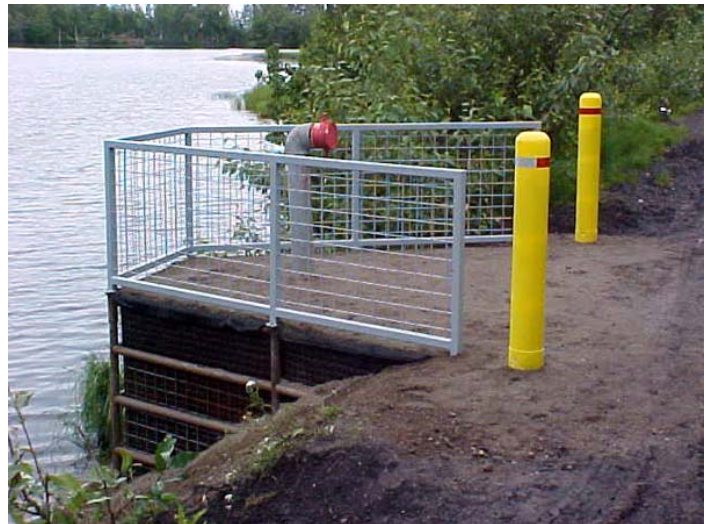
A completed multi-functional stand pipe facility
