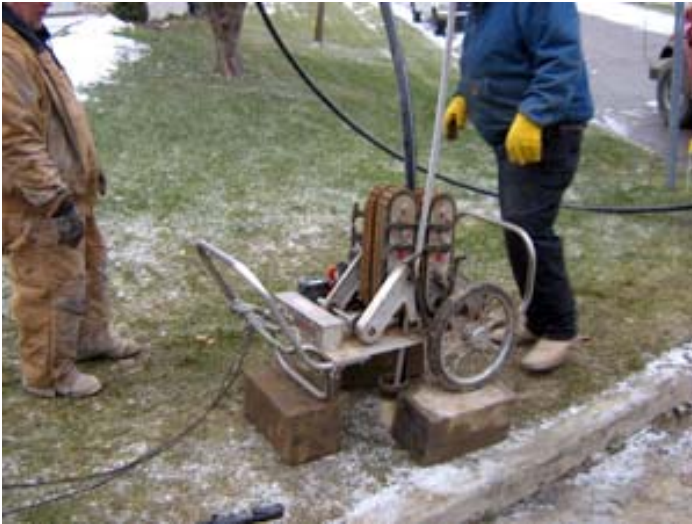
Grouting the borehole
