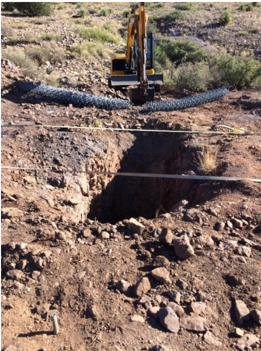
The BLM installing mesh closure at Feature 172094-6
