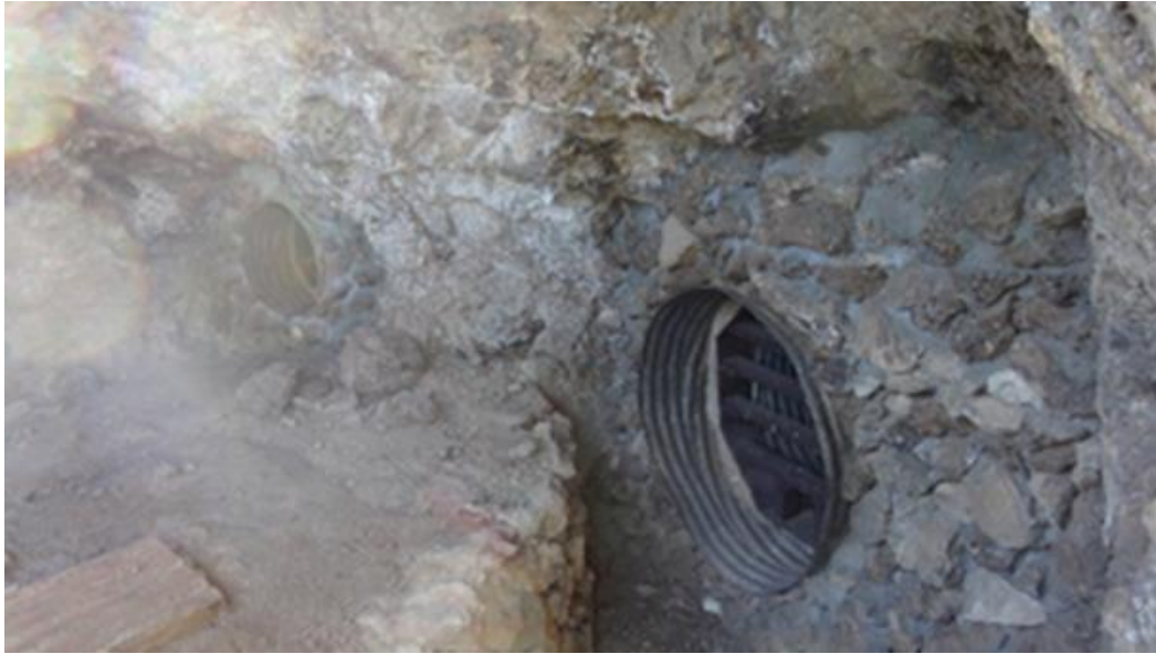
Finished condition of Feature 24
