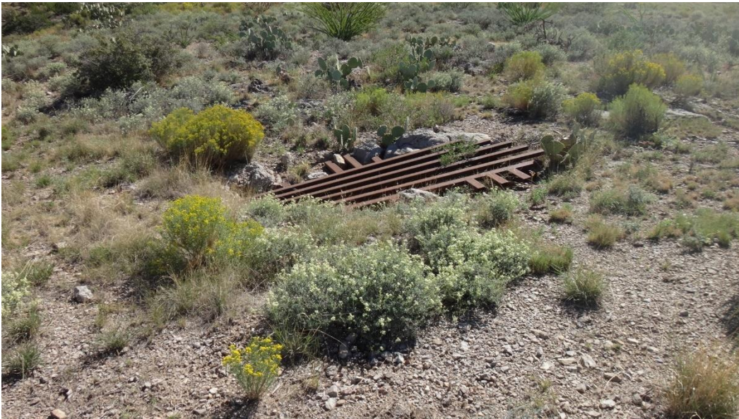
Typical horizontal bat gate that allows for owl use.
