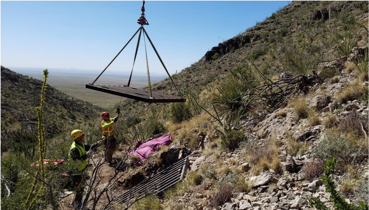
Gate being delivered by helicopter to remote mine shaft.
