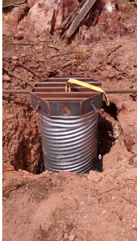
Feature 172095-24: Horizontal Bat Gate being built by the BLM at 100 ft deep shaft.
