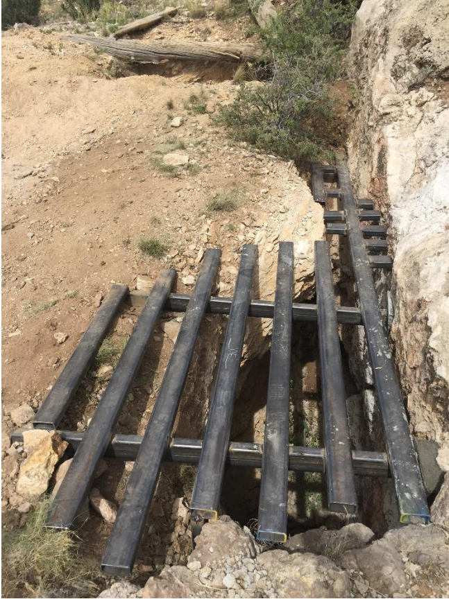
Bat Gate in Rock Bulkhead at Feature 77.
