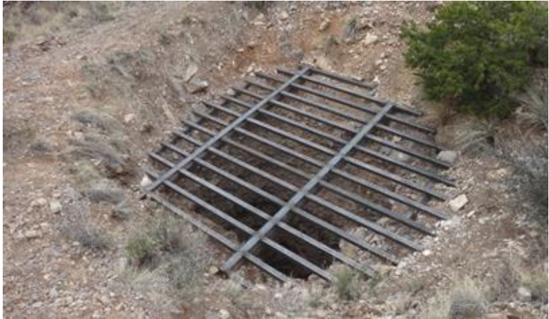
Standard horizontal bat gate installed by Hurricane Industries in a Wilderness Study Area.
