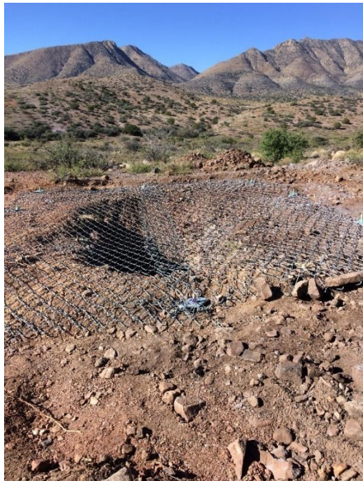
The BLM installing mesh closure at Feature 172094-6
