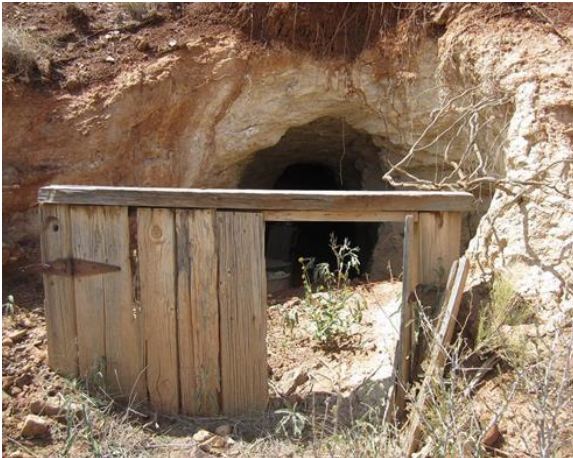
A culvert with bat gate built at Feature 39
