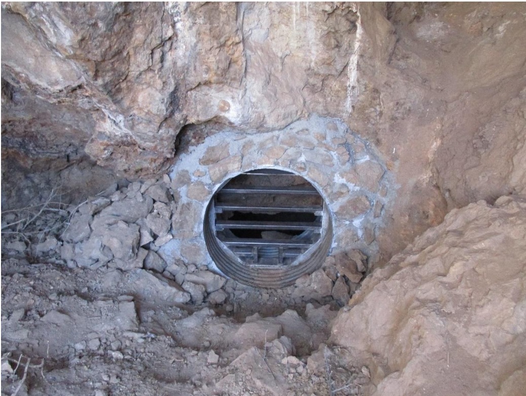
Bat Gate in Rock Bulkhead at Feature 77.
