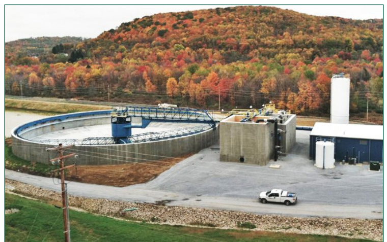
Lancashire No. 15 AMD Treatment Plant
