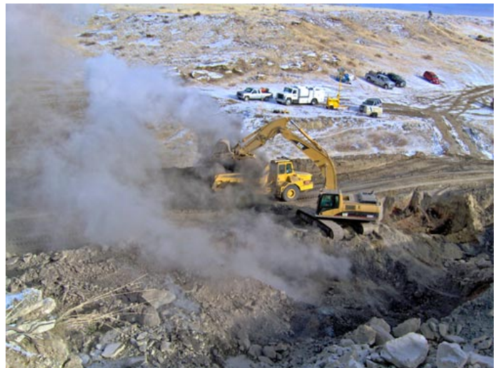
Excavation at the Shepherd Coal Fire
